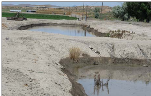
Figure 4. Growers often use tailwater recovery systems with two sedimentation ponds. The first pond is used principally to capture sediment, and the second pond is used principally to provide water storage for stable irrigation.
